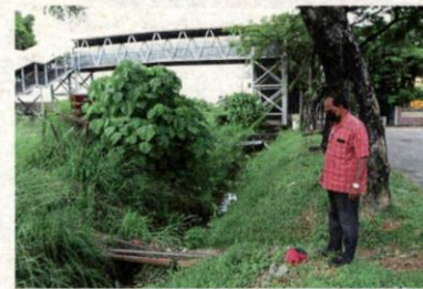
Chandran showing a drain at Jalan Sembilang 8E that is filled with rubbish, silt and overgrown grass. — KK SHAM/The Star
